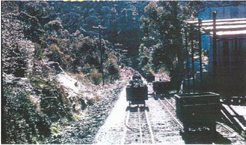
Inclined Tramway at Berrima Colliery showing full skips of coal being raised on the left track and empty skips being lowered on the right track 513
